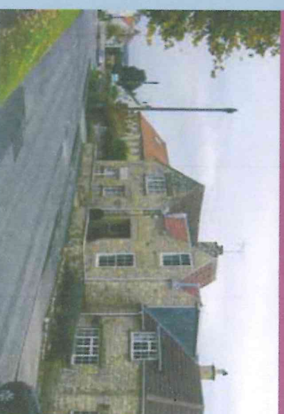
The western gable end of Ivy House Farm clearly showing that part, if not all, of the house was once a single storey structure
