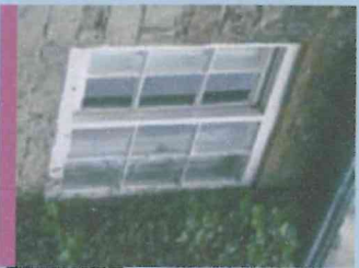
A traditional Yorkshire slider window with wooden frame and glazing bars.
