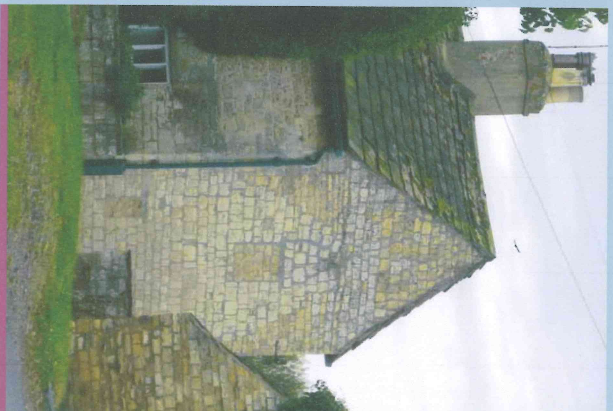
The western gable end of Ivy House Farm clearly showing that part, if not all, of the house was once a single storey structure
